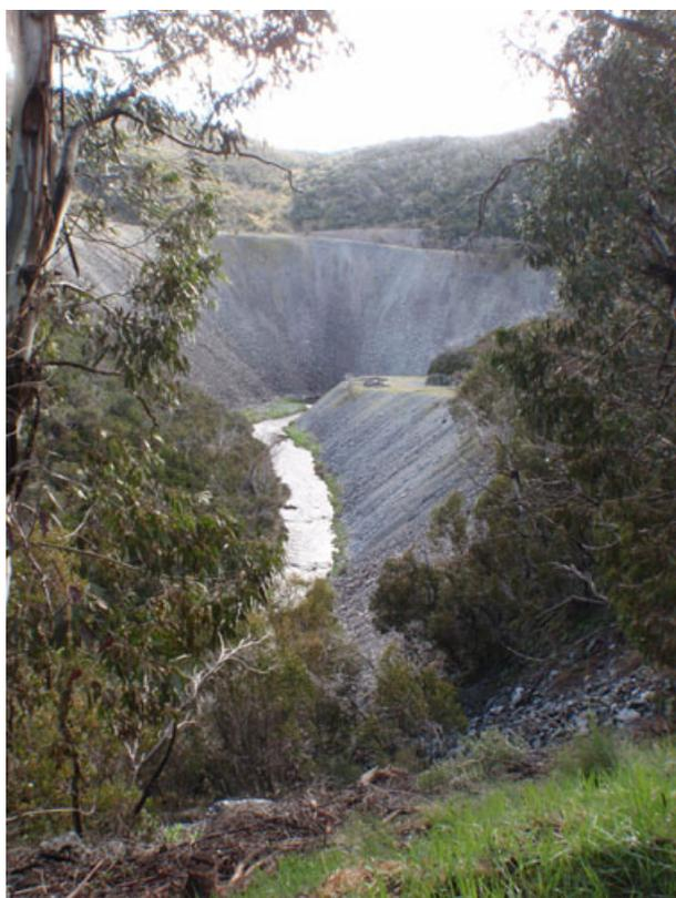
**Figure 3.** Happy Jacks Spoil Dump 1, in which over 970 000 m<sup>3</sup> rock spoil was dumped both sides of the Tumut River, is another of the 35 major sites that has now been subject to rehabilitation earthworks and planting. Its condition prior to treatment, pictured here, illustrates the environmental risk associated with the filling of valleys with spoil rock, which can be further washed down by streams or even block or divert the streams themselves (Photograph Regina Roach).
